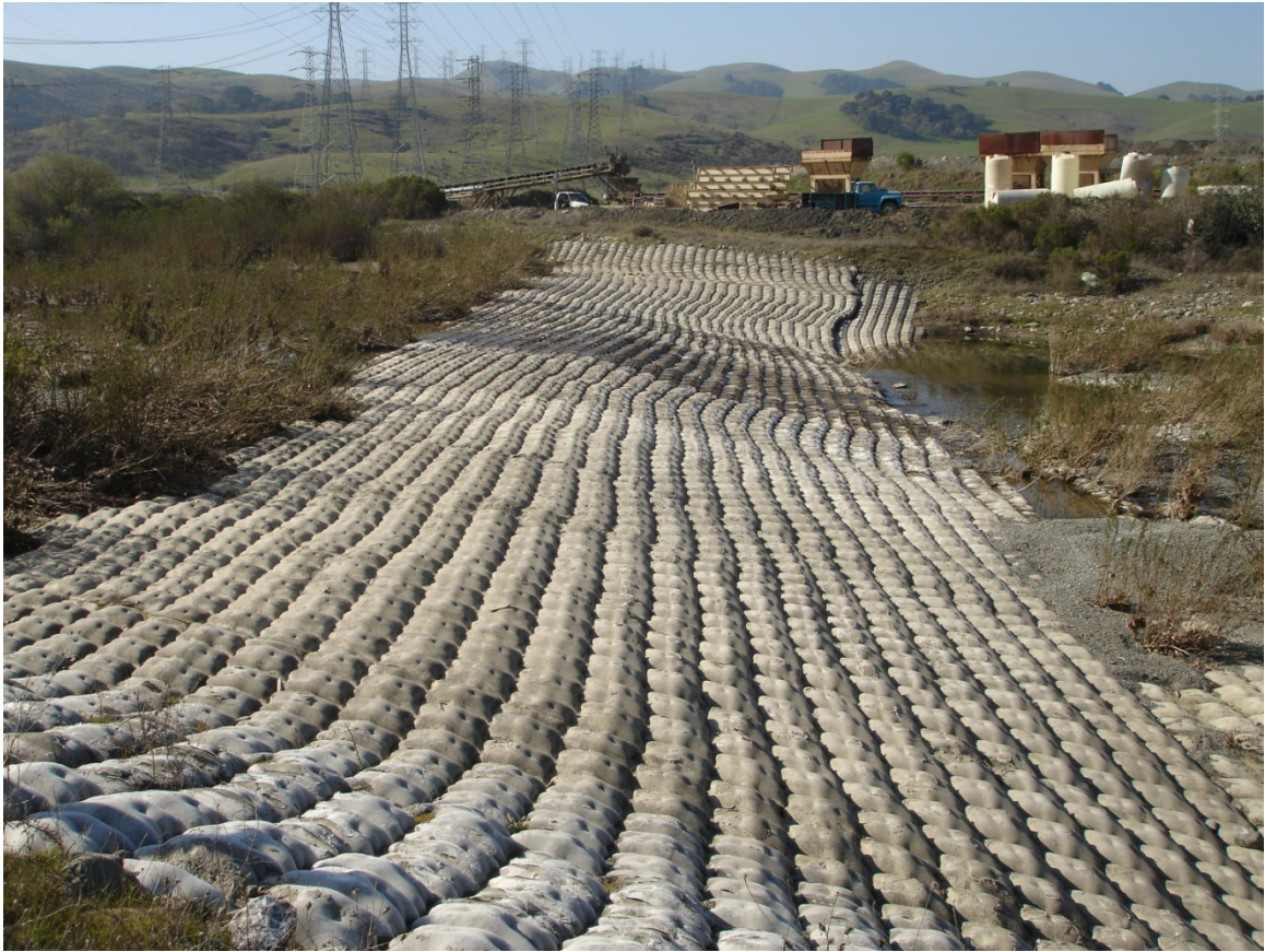
Figure 5-1 PG&E Pipeline Concrete Apron Drop Structure
